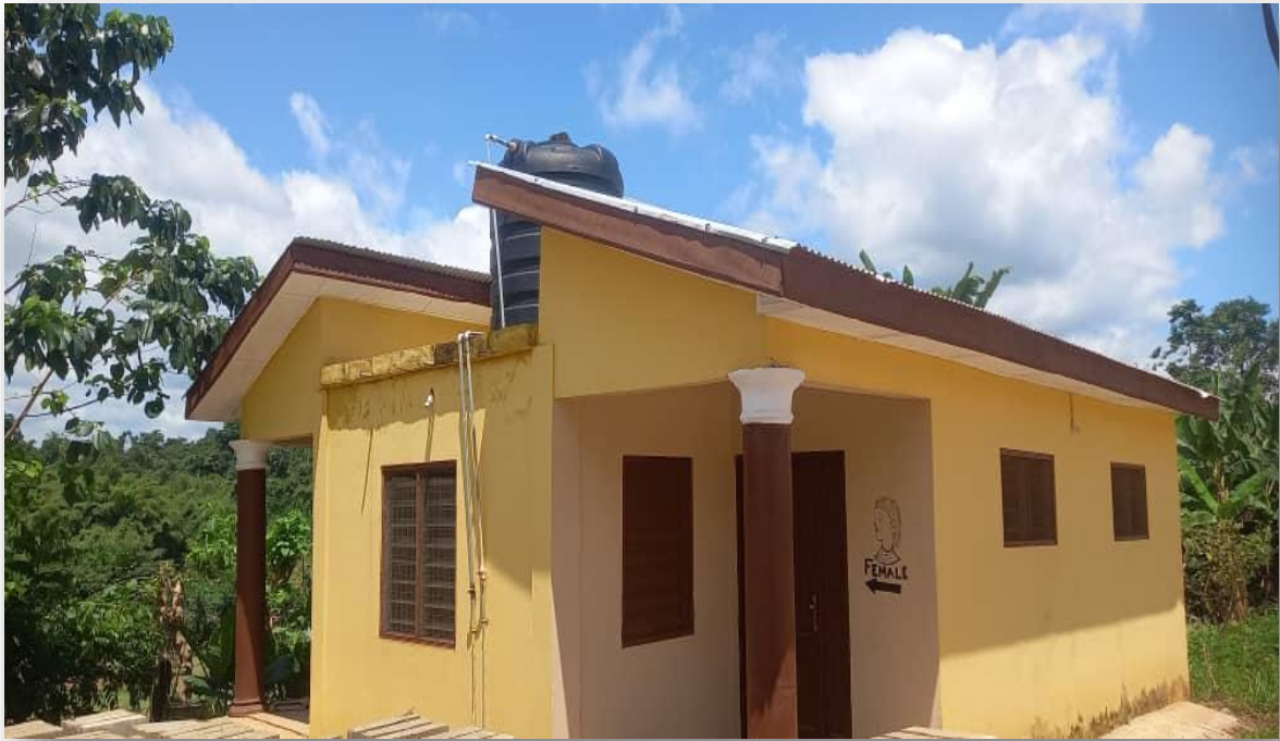
Sanitation: 10-Seater Toilet Facility at Asiwa Lorry Park
